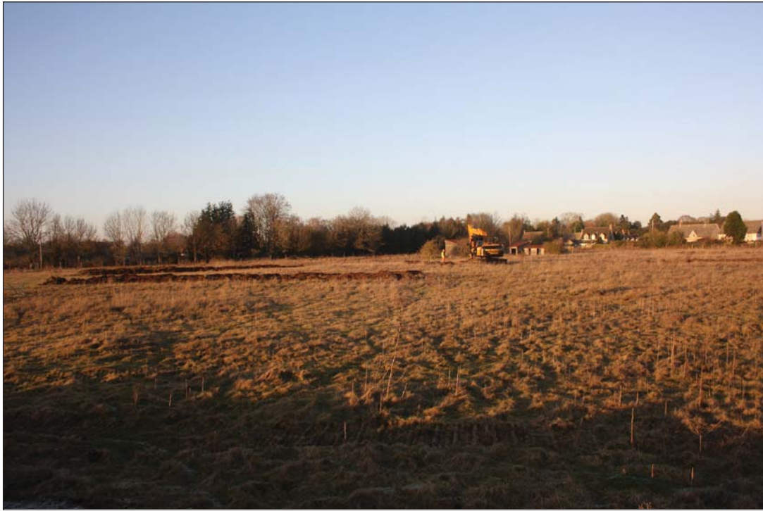
Plate 1: General view of site looking north west.
